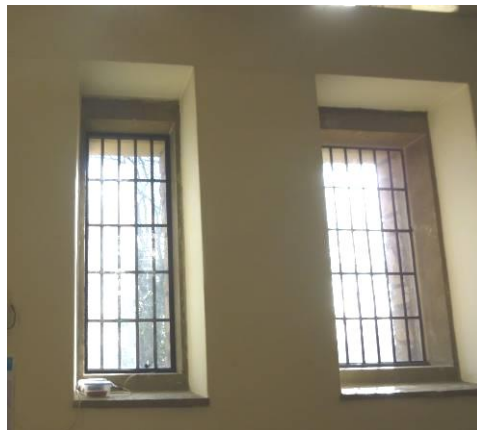
Picture 2: Lower windows with and without double-glazed secondary glazing
