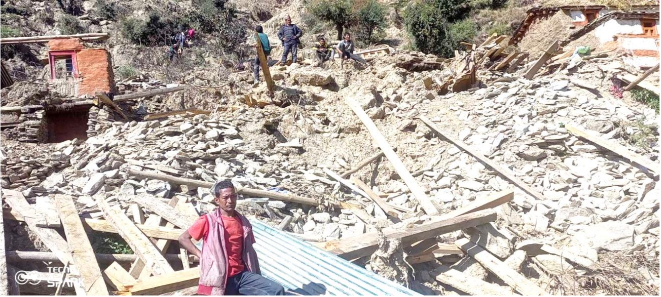
House destroyed by landslide and its owner
