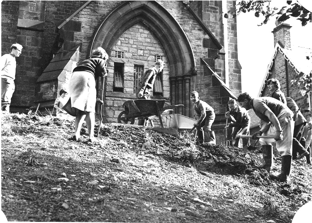
Rebuilding the banking
